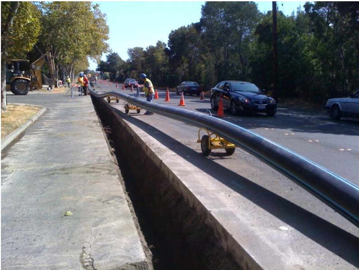
Figure 4. Installation of 12" HDPE by Open Cut
