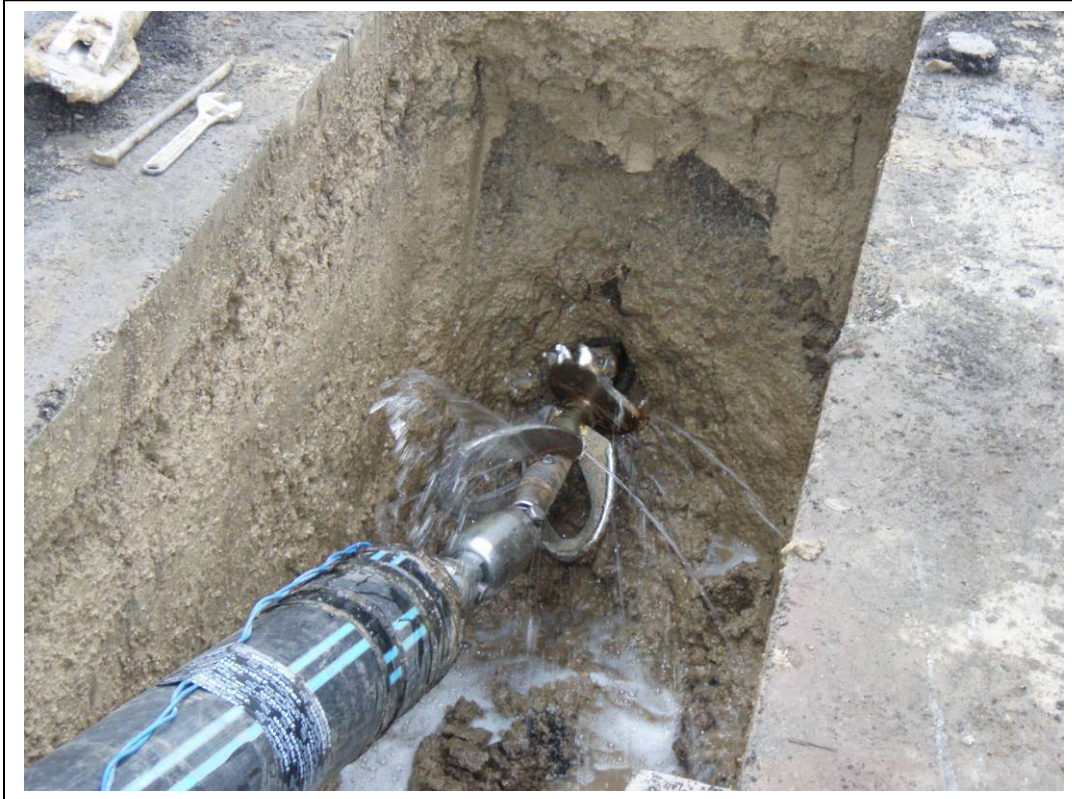
Figure 5. HDD – A borehead in the launch pit.
