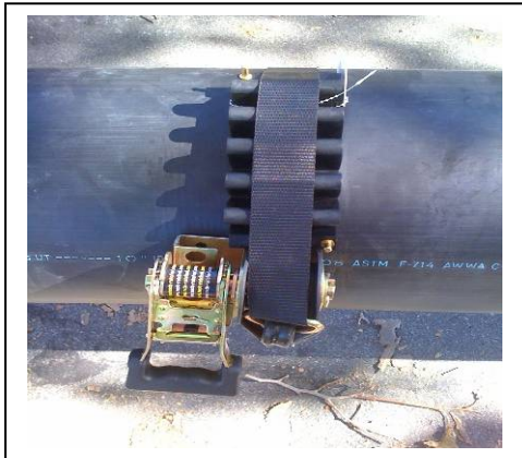
Figure 2. Flex Restraint Installation
