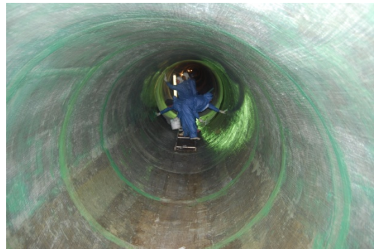
Figure 7(b) Installation of FRP lining
