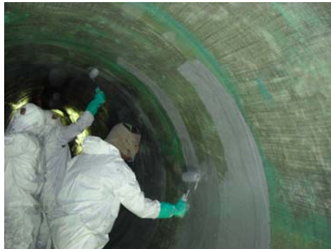
Figure 9: Application of epoxy top coat
