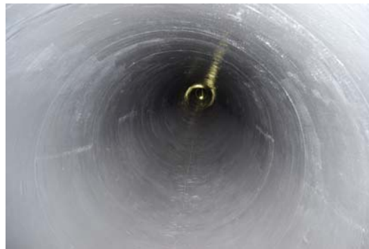
Figure 10: Completed segment of the FRP installation
