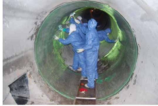
Figure 7(d) Detailing of lining installation
