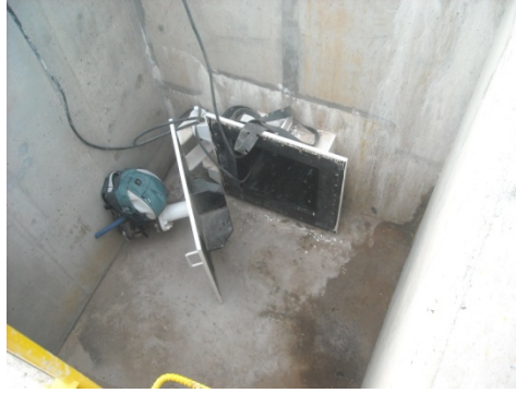
Figure 6: Typical access point
