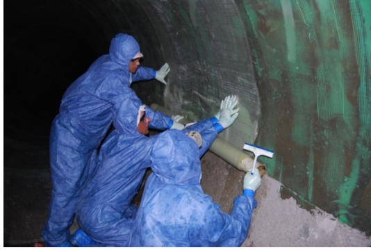
Figure 7(c) Transition between top and bottom half installation
