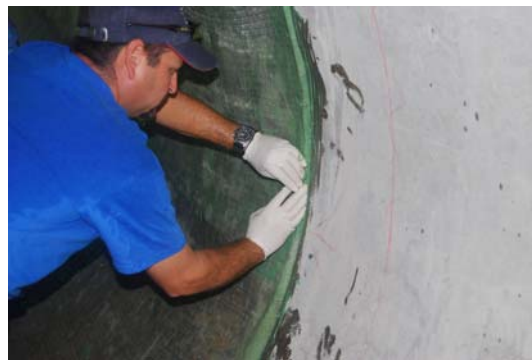
Figure 8: Construction joint of FRP lining
