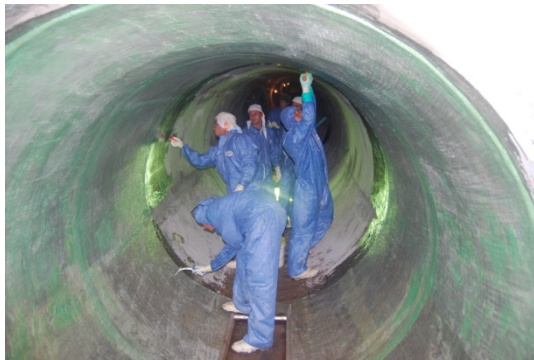
Figure 7(a) Epoxy paste installation on top half of pipeline
