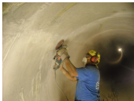
Figure 5: Prep work activities prior to installing FRP lining
