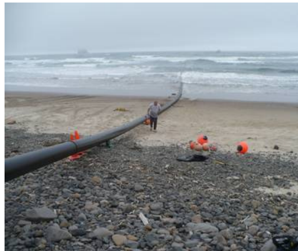
Figure 7. Photographs during product pipe transportation prior to installation
