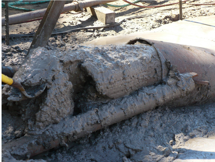
Figure 6. Photograph of clay slugs during reaming process
