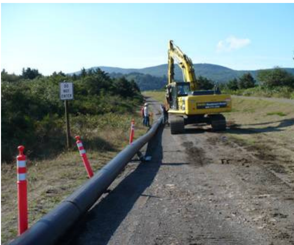
Figure 7. Photographs during product pipe transportation prior to installation
