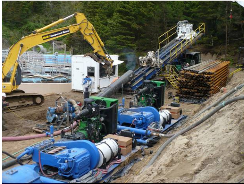
Figure 3. Photograph of staging area next to existing wastewater treatment plant.
