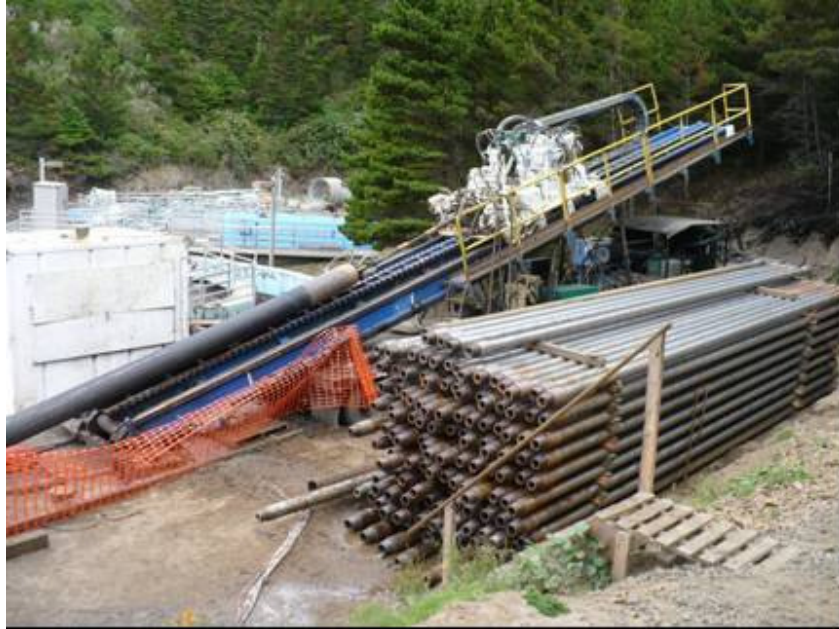
Figure 9. Photograph of completed installation of product pipe
