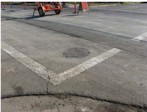
Figure 6. Telephone vault at the intersection of W. 10 th Street and D Street.
