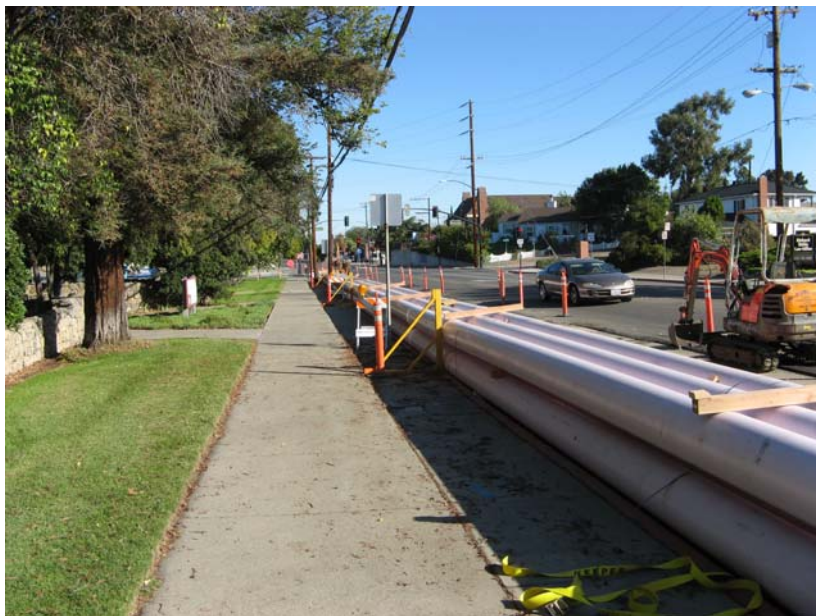
Figure 3. Large laydown area for sliplining procedure near Antioch City Park.
