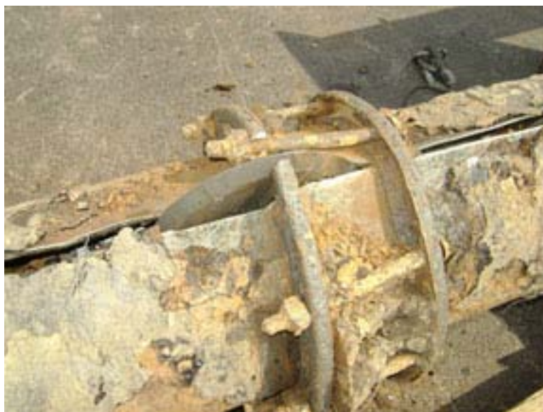
Figure 4. Above ground test, splitting the Dresser Coupling.
