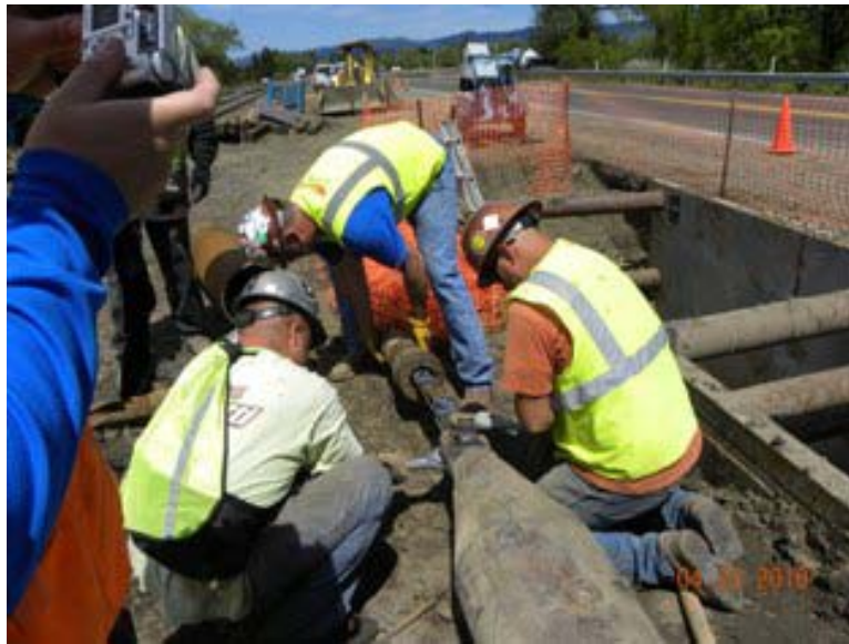
Figure 7. Connecting the bursting head and pipe string.
