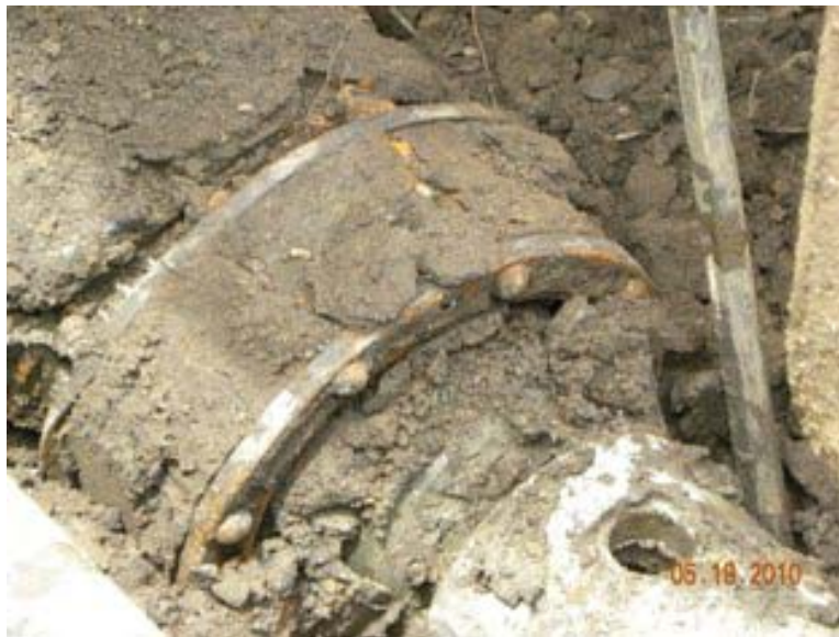
Figure 2. Style 38 Dresser Coupling.
